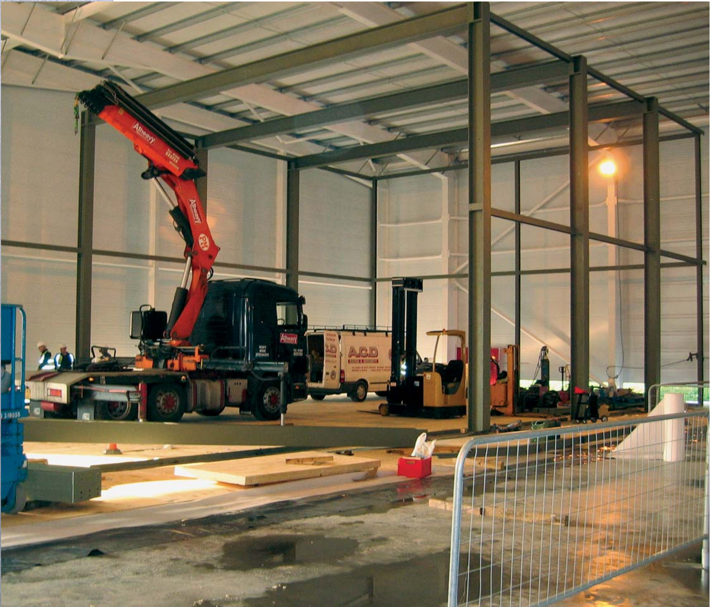
The steel skeleton during construction
